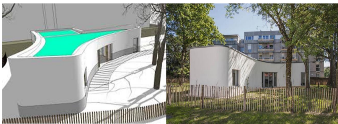
FIGURE 1: Yhnova digital model on the left and the printed house on the right
